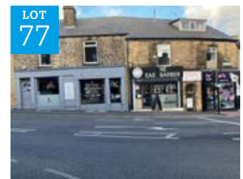
2, 4 & 6-8 Crookes Road/garage At Turner Lane, Sheffield S10 5BB
